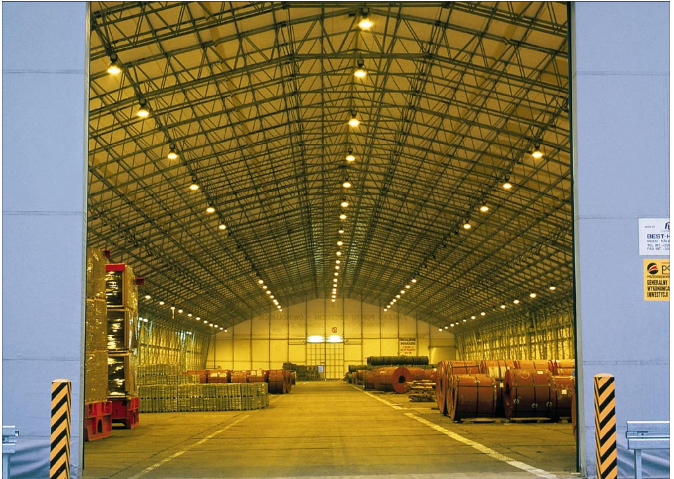
Harbour terminal, 186 x 36 m, 6,696 m 2 Port of Szczecin, Poland.
