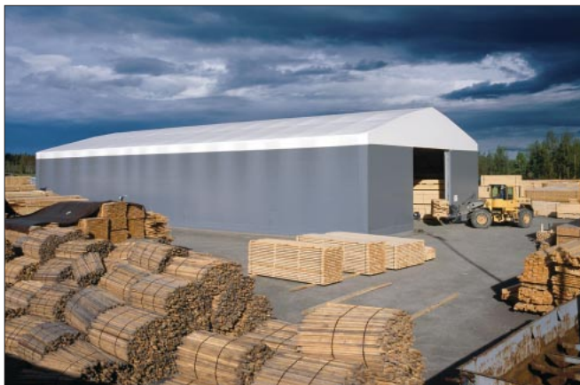
Storage shed 40 x 20 m (800m 2 ) where heat insulation and automatic air dehumidifiers ensure optimum moisture conditions. Mustola Dryer Oy, Lappeenranta.
