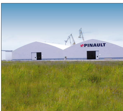
Storage sheds for timber, total 4,800 m 2 . Pinault SA, Honfleur, France.
