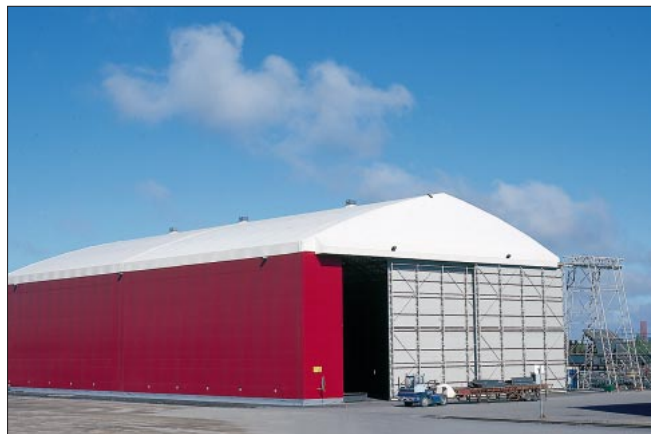
Production facility for metal industry. Hall's lowest free height 15 m, size of sliding door 30 x 15 m. Aker Mäntyluoto Oy, Pori.
