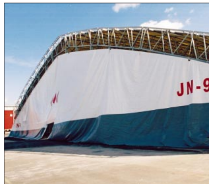
The end walls' fabric is lifted and attached to the frame.
